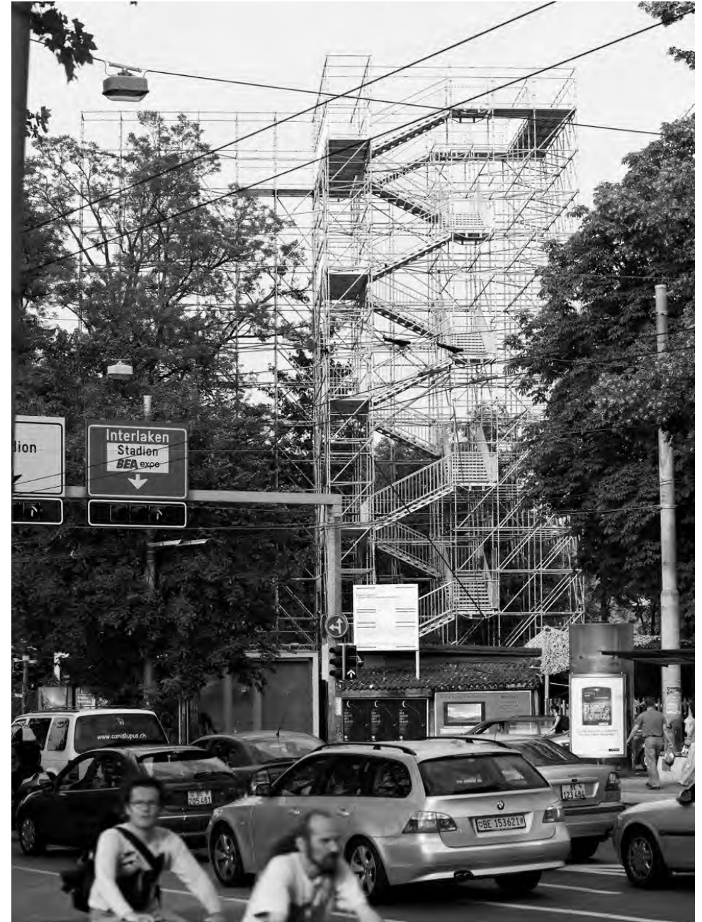
The 25-metre scaffold tower rising beside the Lorraine Bridge. Photo: David Aebi.
