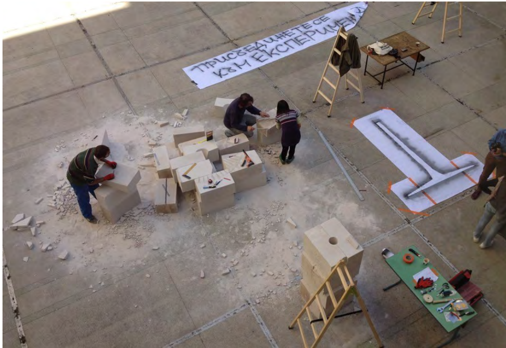
Production view: building the clay-and-straw column in the courtyard of the university. Sofia, 2013.
