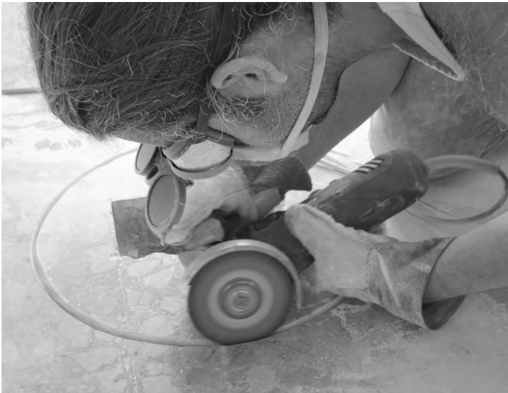
Production view: cutting the openings with an angle grinder. Rome, 2005. Photo: Jürg Orfei.
