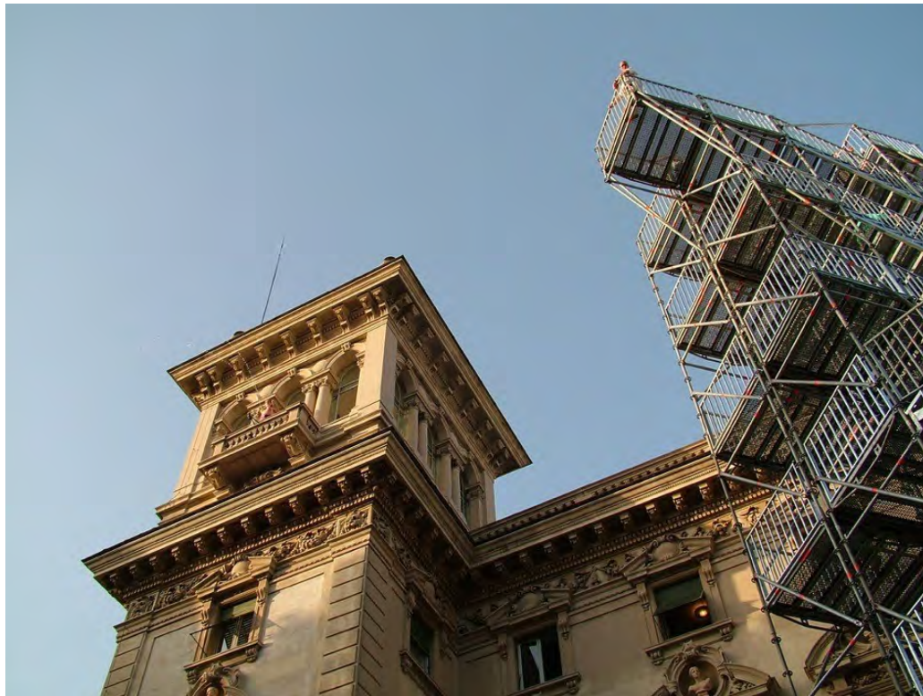
The walkable scaffold frame on the garden façade of Villa Maraini. Photo: Markus Rottmann.
