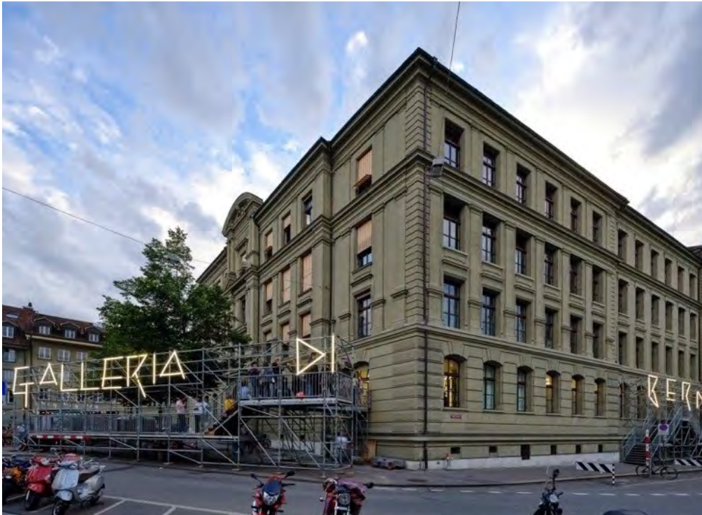
Scaffolding and light installation in front of the Stadtgalerie, reading 'Galleria di Berna'. Bern, 2021. Photo: David Aebi.
